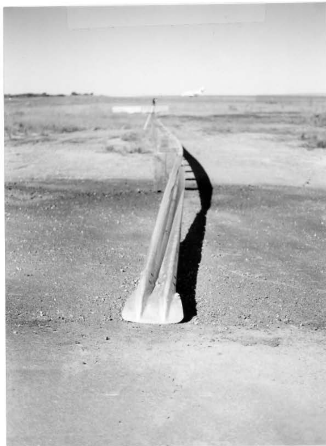
FIGURE 27. Turned-Down Terminal Anchored Above Grade with Michigan End Shoe
