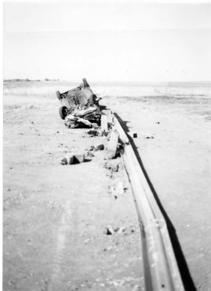
FIGURE 31. Guardrail Damage
