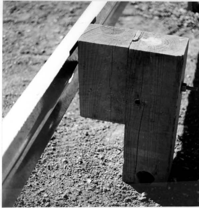
FIGURE 22. Post, Blockout, and Backup Plate Configuration.
