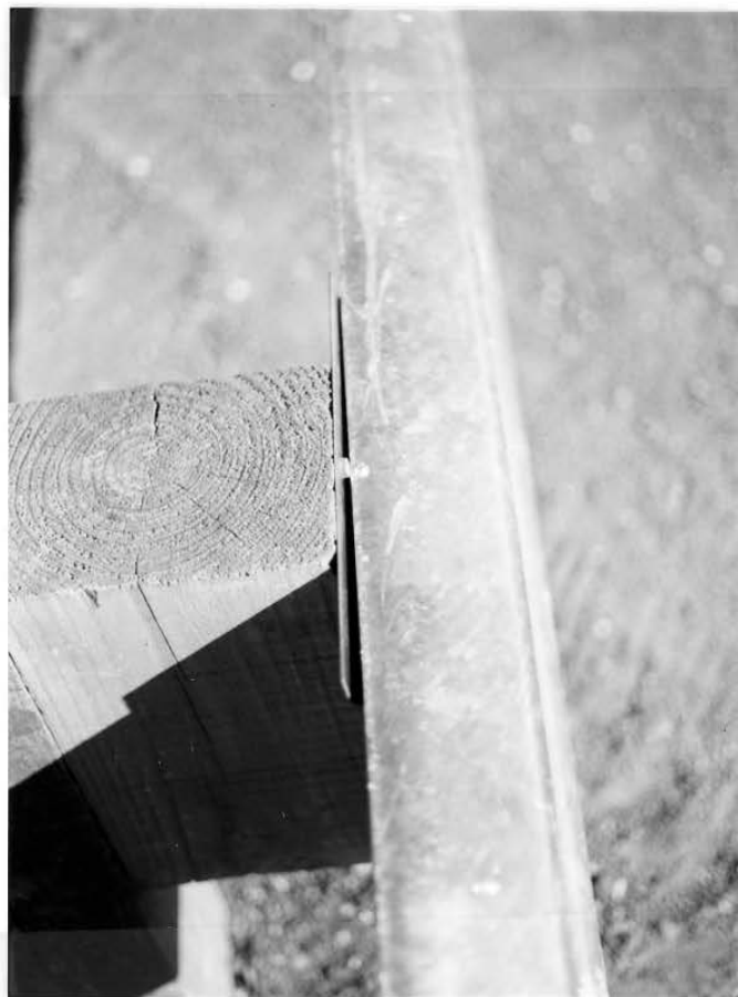
FIGURE 23. Guardrail-to-Backup Plate Connection.
