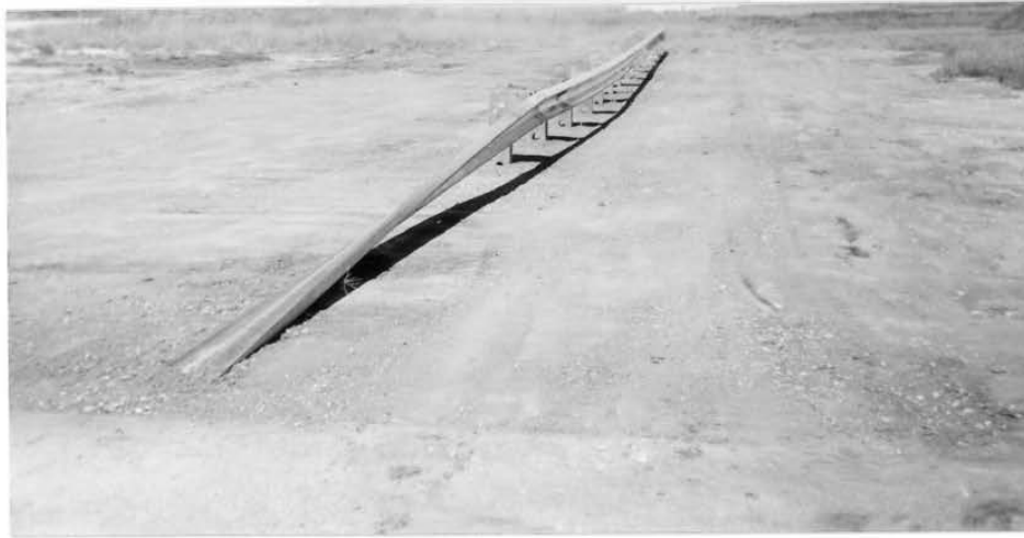
FIGURE 26. Turned-Down Terminal Section with 90 deg CW Twist.
